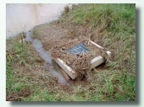
Pond outlet blocked with debris
