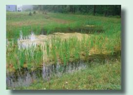
This is a poorly-constructed pond because it is too shallow to function properly
