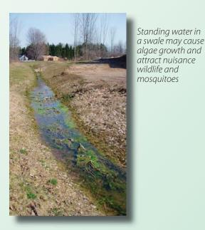
Major repairs to ponds and swales must be done by a professional.
