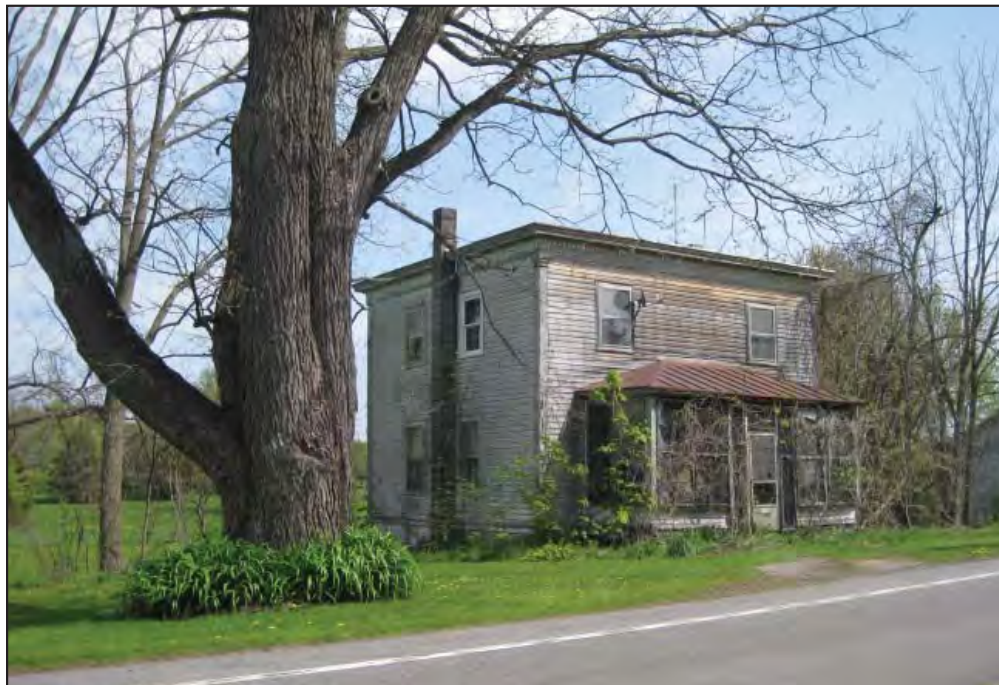
At left, an old house in the Hamlet of Victory is just one example of the many historic resources in the Town that should be documented and preserved where possible.
