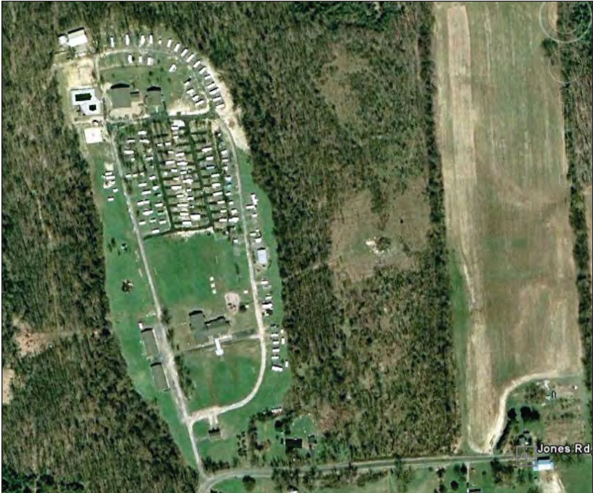
Northeast Christian Center camp and conference center located on 107 acres on Jones Road
