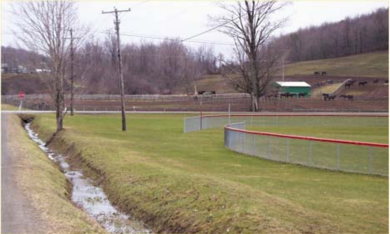
Figure 7. Ditch that runs into a culvert at site 16. Note extensive area of exposed soil in pasture of grazing horses.
