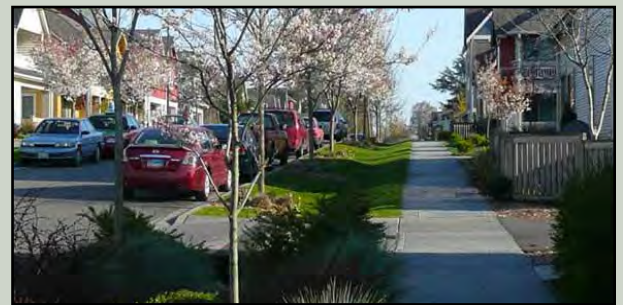
Bioretentions are landscaped depressions designed to slow and treat stormwater runoff. They are often used in parking lots and residential areas. (Source: http://www.tataandhoward.com/tag/stormwater-management/ )
