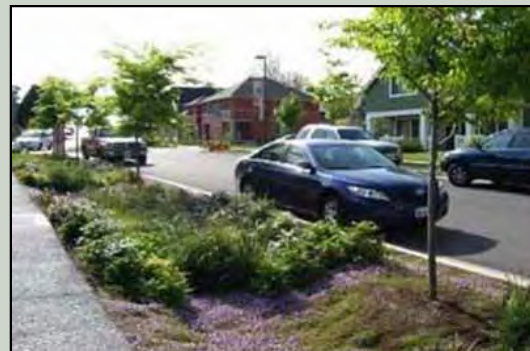
Vegetated swales slow, infiltrate, and filter stormwater runoff. They are well suited along streets and parking lots. (Source: http://www.3riverswetweather.org/green/green-solution-vegetated-swale )
