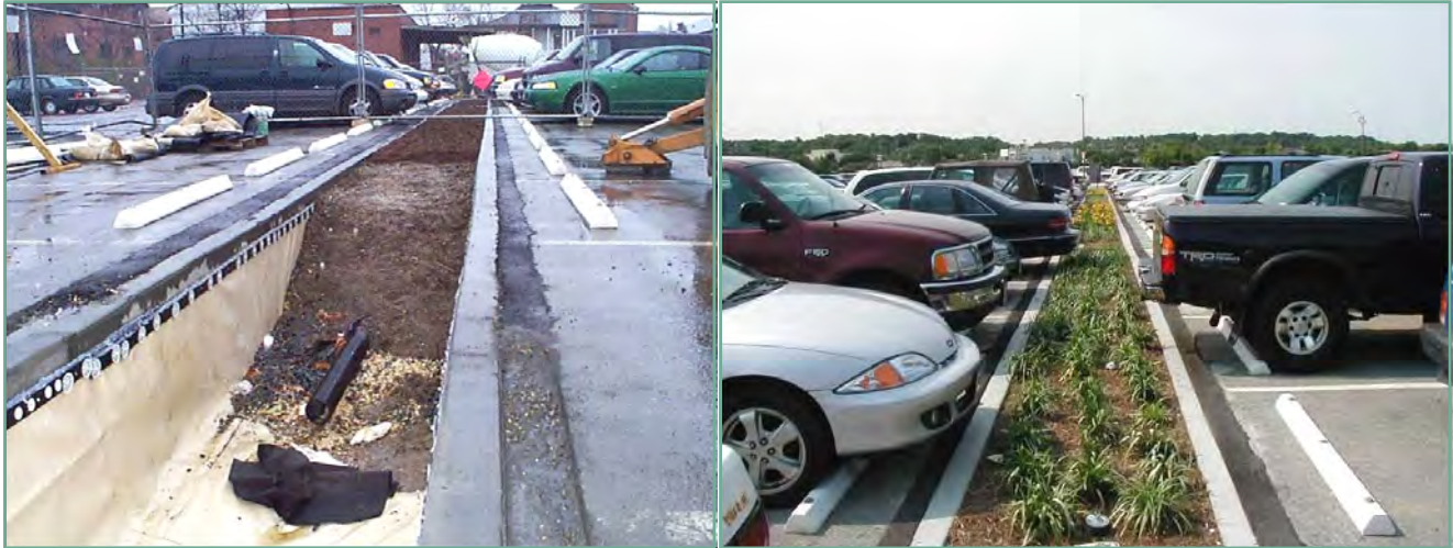
A bioretention area under construction (left) and completed (right).
