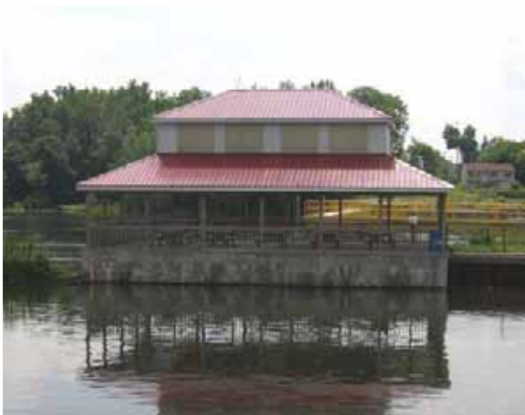
A photo of the gazebo located on Lock Island.
