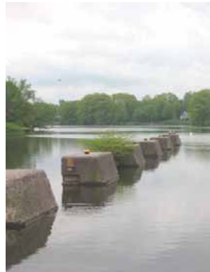
The installation of floating docks alongside these concrete impoundments is one recommendation of the VRC.
