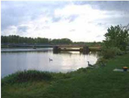
Oswego River Canal in the Village of Phoenix.
