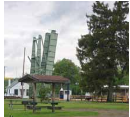
The drawbridge at Lock Island Park.
