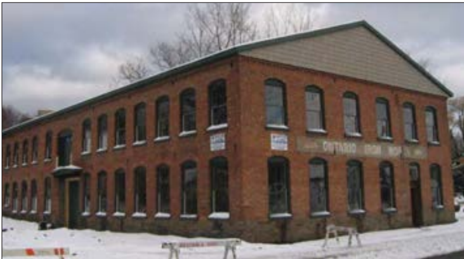
The Ontario Iron Works Foundry Building on Maple Avenue in the Village of Pulaski.
