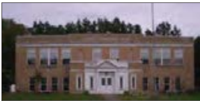
Half-Shire Historical Society building in the Town of Richland.
