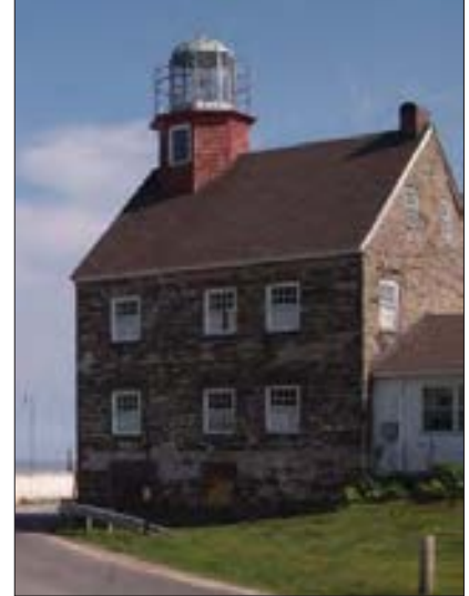
Selkirk Lighthouse, Summer 2008.
