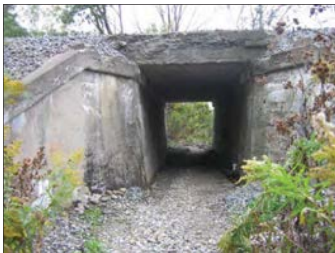
An existing railroad underpass could be improved to provide a safe link for bicycle and pedestrian use between Rome Road and the Salmon River Greenway Trail.
