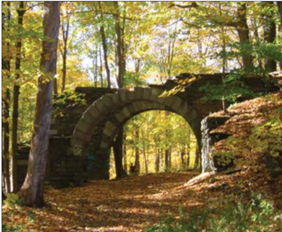
Remains of the Syracuse Northern Railroad arches in the Village of Pulaski.
