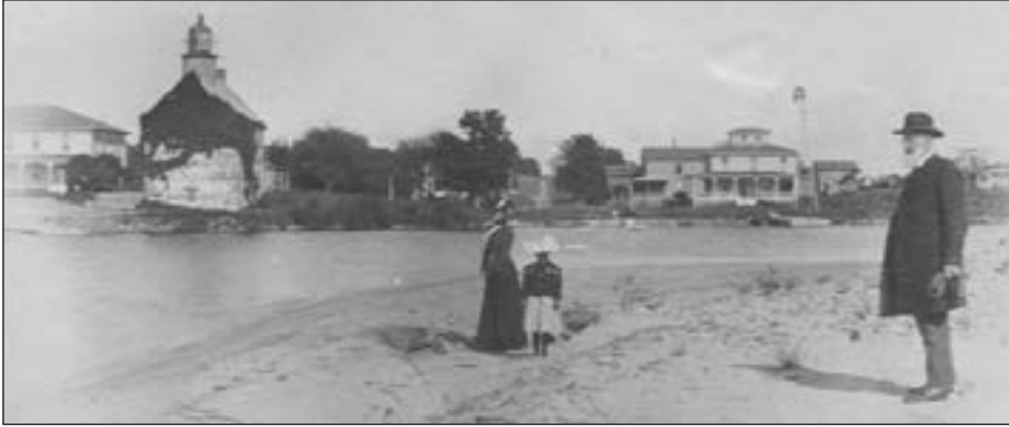
Selkirk Lighthouse Spring 1902. Source: www.rootsweb.ancestry.com/~nyoswego/towns/richland/photo5.html , contributed by Julie Robst.
